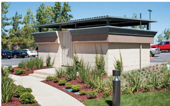
Trash enclosure: In keeping with the practice’s high curb appeal, contractors built the trash enclosure to match the hospital’s architecture. One bioswale sits to the right of the enclosure. A hospital design competition judge commented, “That’s the nicest trash enclosure I’ve ever seen.”
